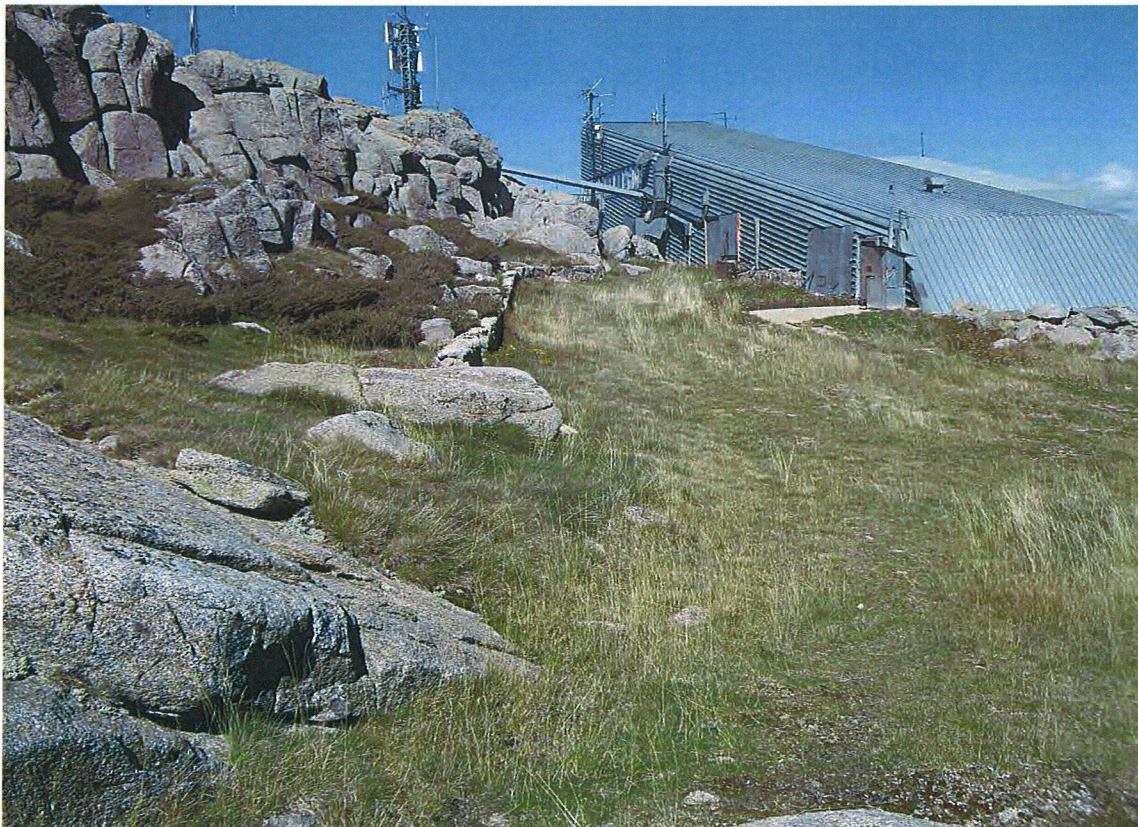
Photo 3: Disturbed area where the services trench will be located between the communications hut and the Eagles Nest building.
